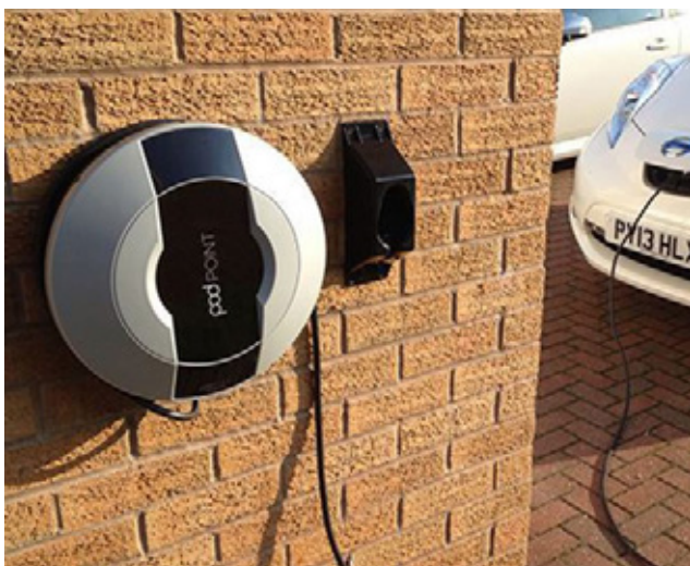
Figure 58: EV charging point
